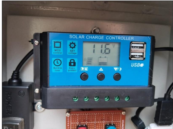
Gambar 3.16 Solar charger controller
